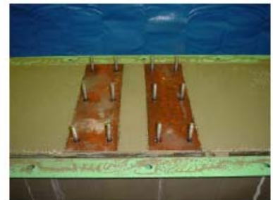
(c)H型鋼周辺の充填状況
