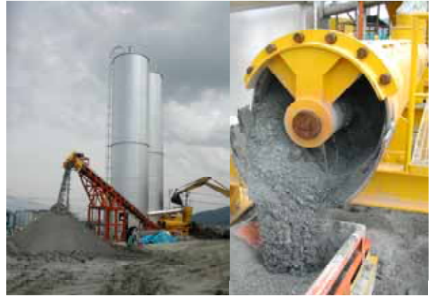
Photo.5 Improvement system of lacustrine deposit
